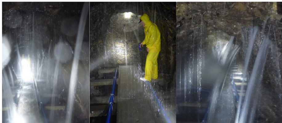
Fig. 4: Impressions from the interior of the Muehlau spring tunnel system. The capture gallery has been set within the saturated zone. The water enters from numerous open fractures and is collected in a rectangular channel and transported outwards (Photos: R. Benischke, G. Winkler).
