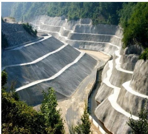
Fig. 2. Insulation of the bed of Gashnia River
