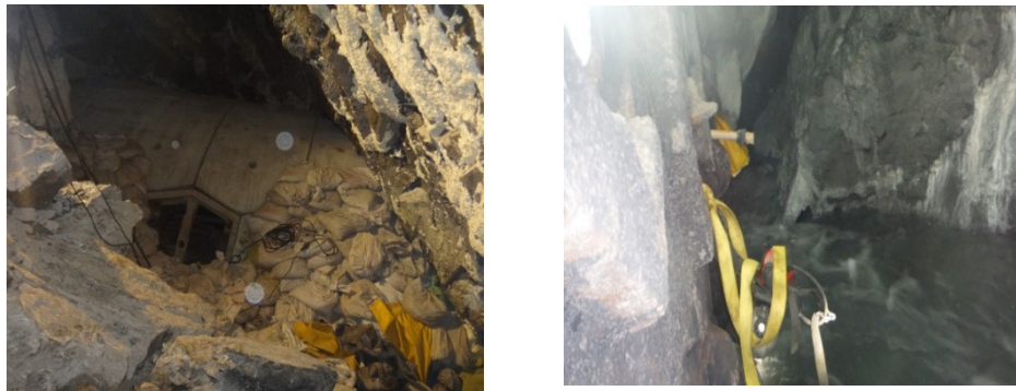
Fig. 5. Right-F16 Fault Area 19632 - Left Hollow Area 19672- Empty Space behind Segment- Stone: Brecciated Dolomite
