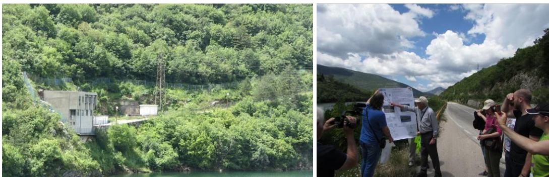
“Oko” tapping structure
